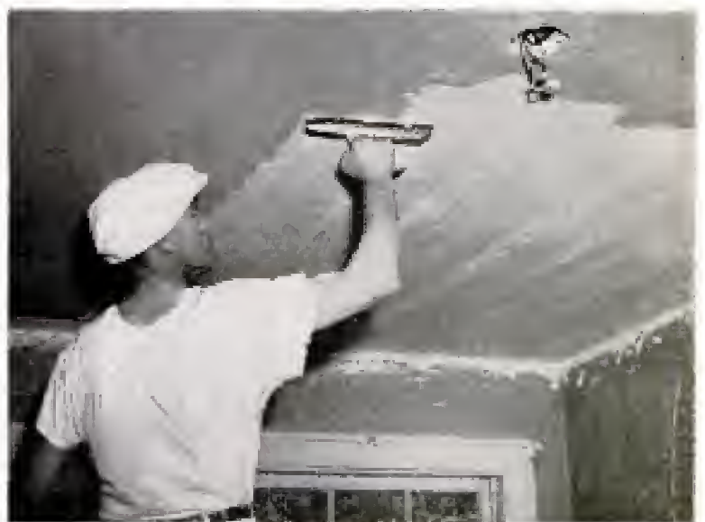
Finish coat can be applied 24 hrs. after base coat. Photo above shows start of finish-coat application, beginning at side of room and working toward center
